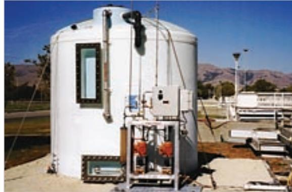
*Trojan UV-oxidation solutions include complete H<sub>2</sub>O<sub>2</sub> storage, delivery and monitoring systems that meet the most stringent safety standards.*
