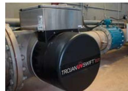
**Figure 2.** The City of Cornwall, Ontario, Canada currently uses the TrojanUVSwift™ ECT to provide year-round primary disinfection and taste and odor removal during intermittent T&O events with a design flowrate of 26.4 MGD (4,164 m<sup>3</sup>/hr).
